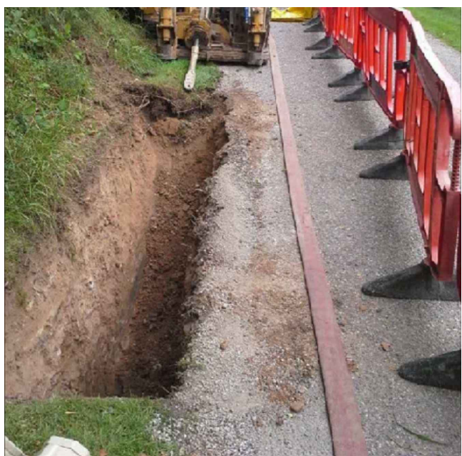
TYPICAL DRILLING RIG & LAUNCH PIT
